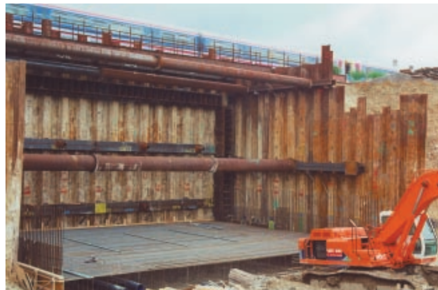
The near completed view of the total 82 'I' beams installed.
