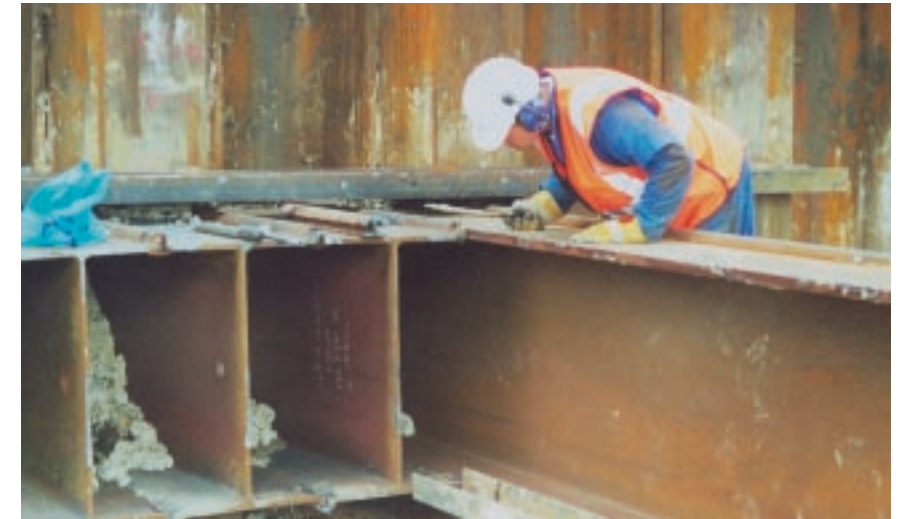
Each 'I' beam installed was carefully aligned using interlocking steel profiles.
