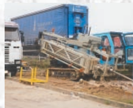
The GRUNDODRILL 20S in action.
