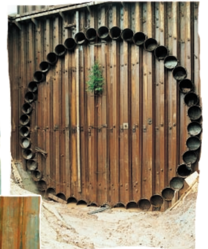
◀ 180 Dywidag threaded steel connections were used to stabilise the embankment.
