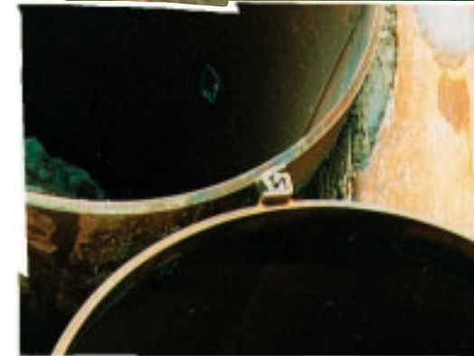
For exact alignment interlocking steel profiles were welded on each pipe.
