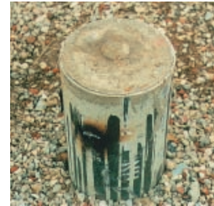
The steel pipe, already advanced and filled up with high-quality grouting mortar.
