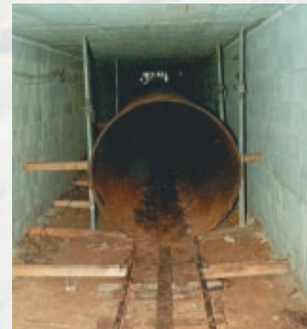
The entrance of the tunnel was very cramped.
