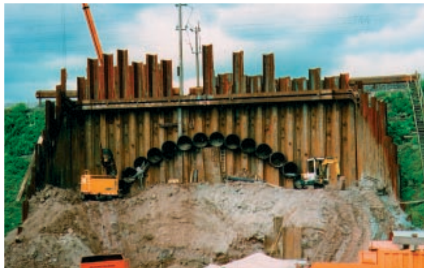
The initial view of the tunnelling project.
