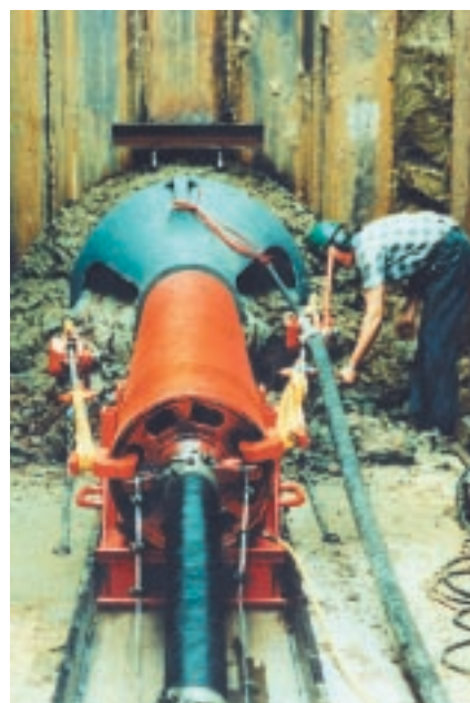
Soil removal cone for automatic removal of the soil during propulsion (partial removal during propulsion).
