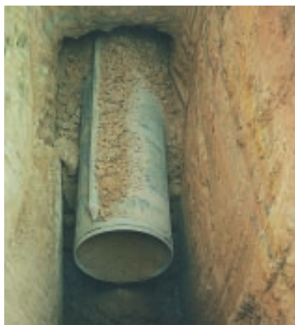
View of the steel pipe after soil removal.
