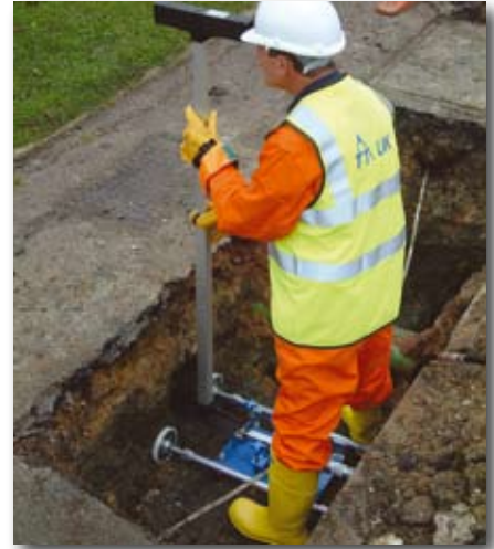
Driven with compressed air (compressor 7 bar).
