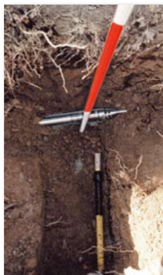
Producing a service connection.
