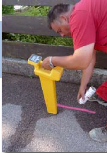
Location of adjacent service pipes/cables.
