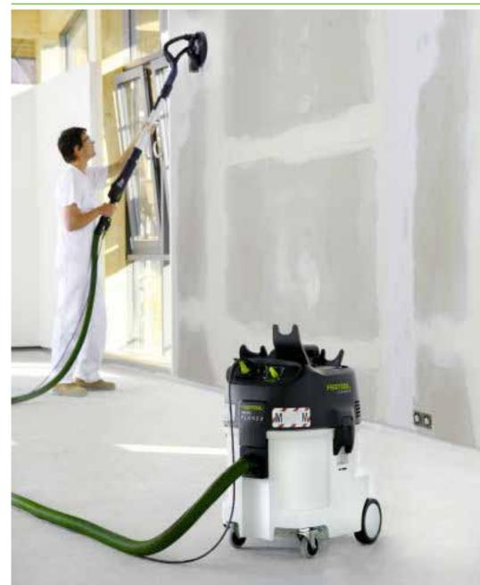
Extraction with system – for extracting fine dust over large surfaces.
