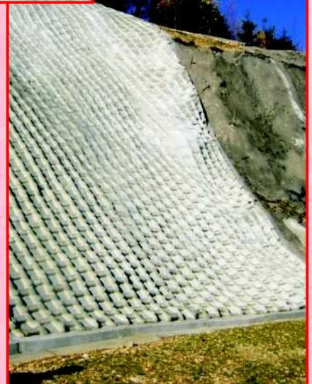
*In the shortage geomorphologic conditions company Züblin Romania executes slope protection for buildings with different importance, against versant slides. Is used for protecting the acclivities of the excavations for communications paths modernizations or on segments where the existing protections were deteriorated.*
