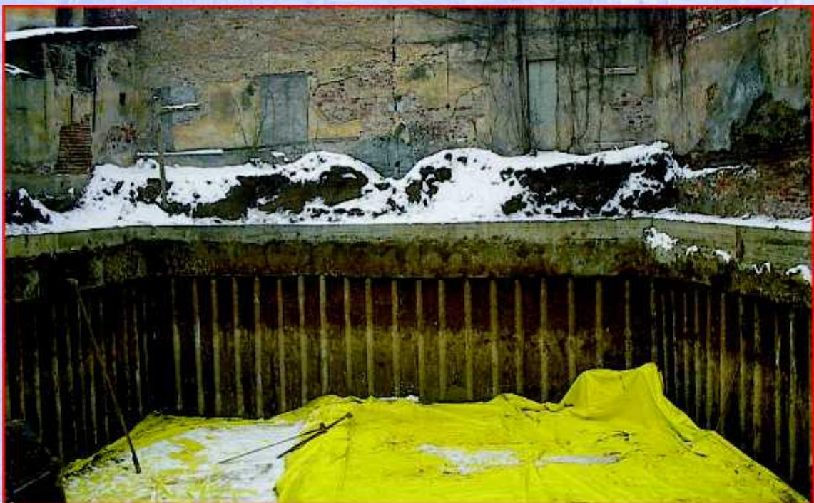
*"Berliner verbau" is a provisional work to prop up of enclosures or the slopes, and can be used only in the conditions which the hydrostatical level is below ultimate quota of excavation with at least 50cm.*
