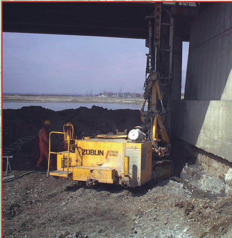
*Züblin Romania executes minipiles at any inclination including horizontally in all category of soils, cohesive or not, upon or beneath the water table.*
