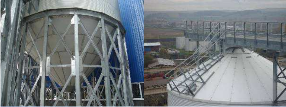
Romania – 4 silozuri 840/13T/45 , 2 silozuri 760/11T60
