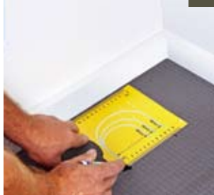
Measure out the required cable spacing
