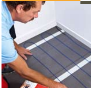
Install the cable
