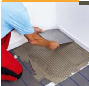
Install the tiles
