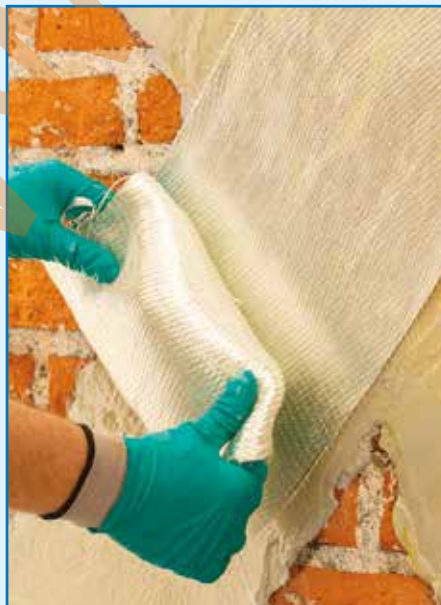
Application of MapeWrap G UNI-AX fabric
