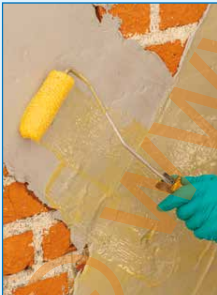
First coat of MapeWrap 31
