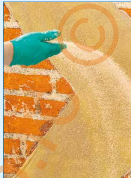
Broadcasting of quartz sand
