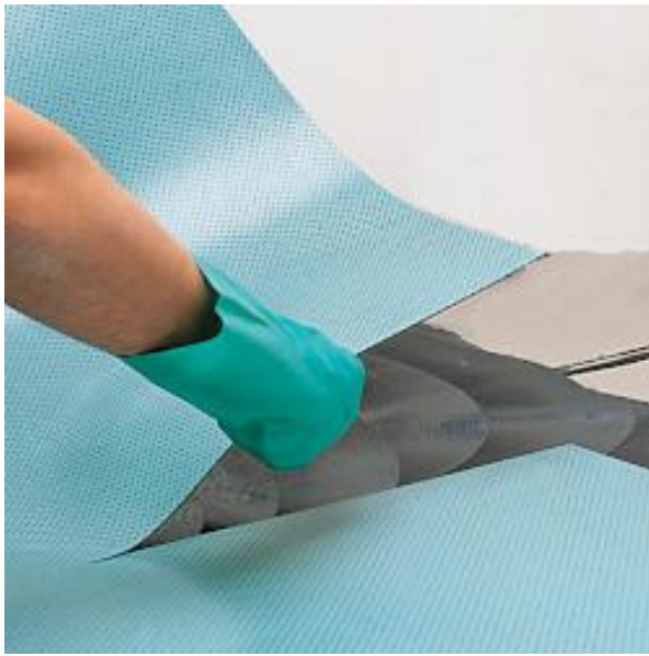
Laying conductive PVC tiles
