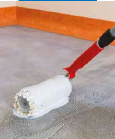
Application of Eco Prim T Plus with a roller
