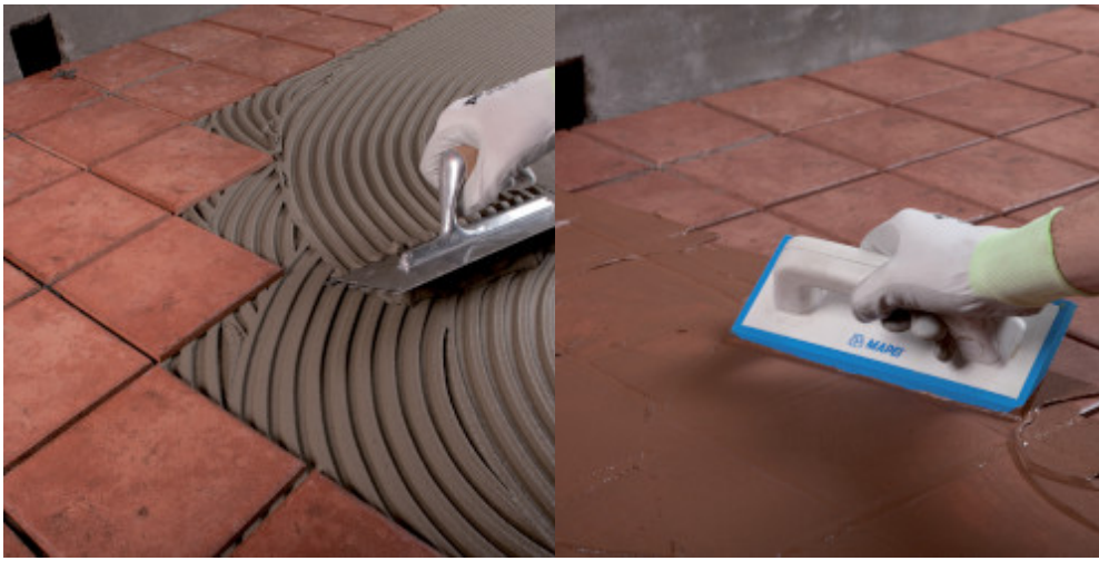
12. Bond on the skirting boards and grout the vertical joints
