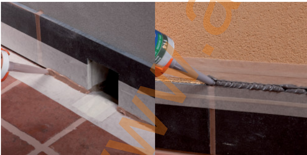
13. Seal with Mapesil AC in correspondence with the skirting board-wall fillet joint
