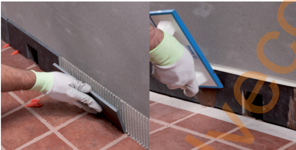
13. Seal with Mapesil AC in correspondence with the skirting board-wall fillet joint
