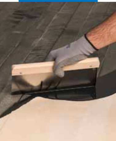
Application by trowel with Ultracoat Steel Spatula
