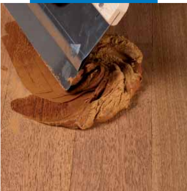
Mixing of Ultracoat Binder
