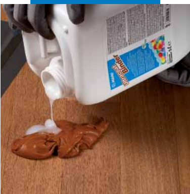
Mixing of Merbau powder with Ultracoat Binder
