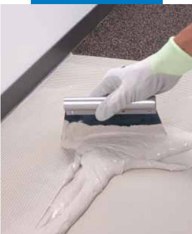
After suitable preparation of the substrate, spread on the adhesive to bond the soundproofing sheets
