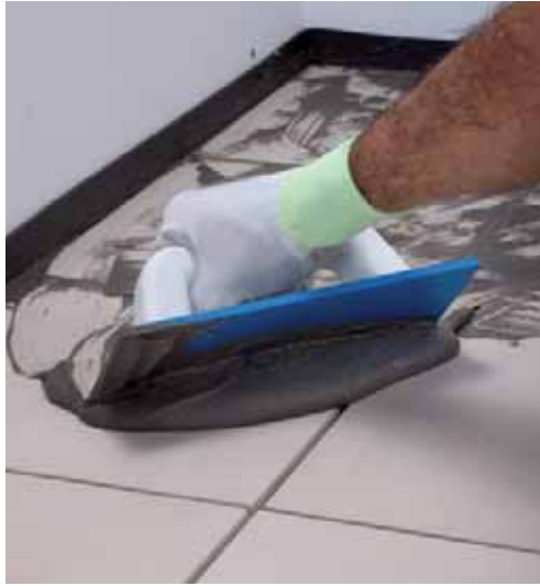
Grout the surface of the room
