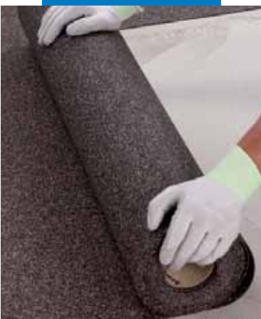
Unroll the sheets of Mapesonic CR on the surfaces to be soundproofed
