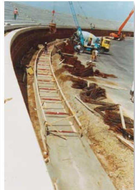
Aluminium panels as formwork for a pocket foundation
