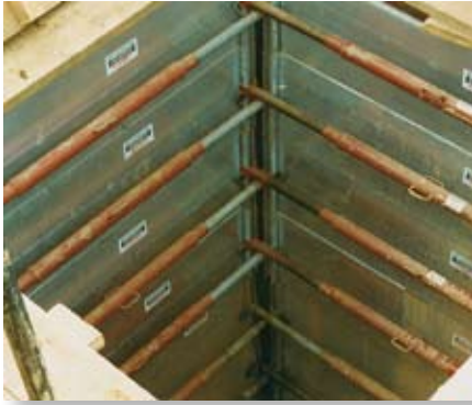
Special solution: manhole lining with additional struts
