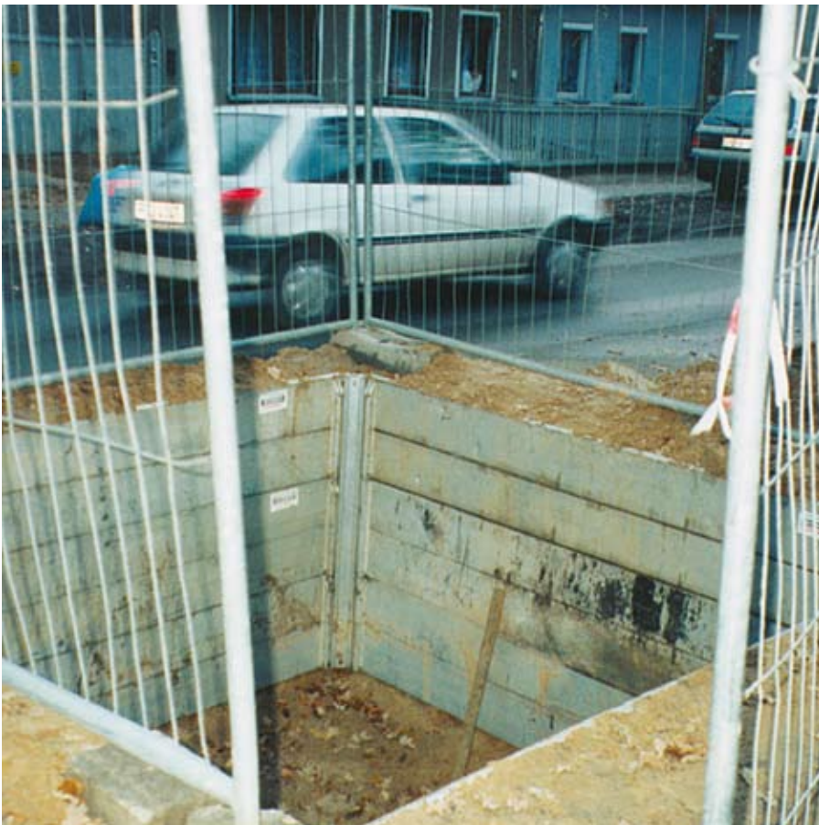
Renewal of road gullies
