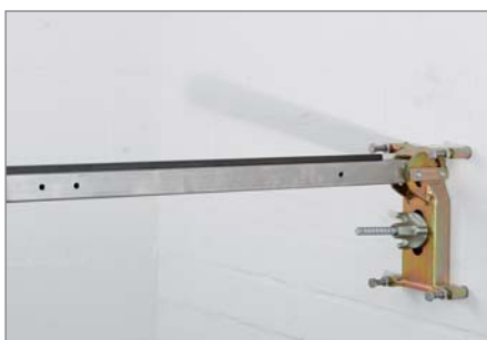
fixing the dowel foot with the column to the wall
