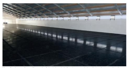
View of an intermediate ceiling made of plastic boards before the system is installed on the second level
