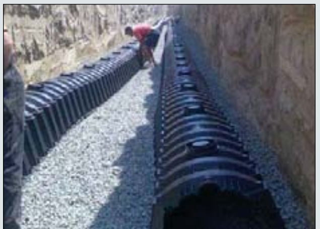
Infiltration system with GRAF infiltration tunnel, Galati (RO)
