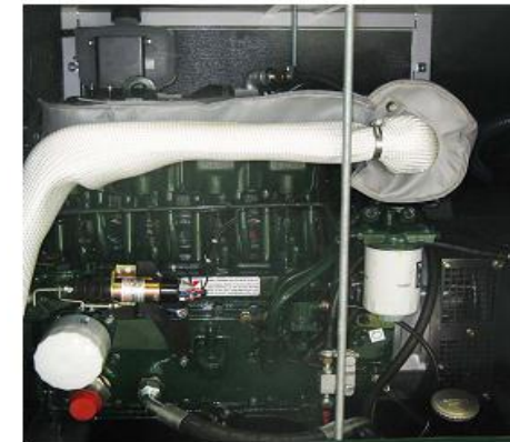
DETAIL OF INTERIOR
